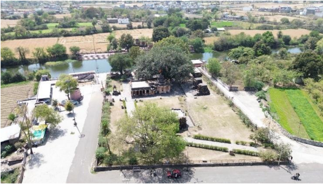
Figure 31 An aerial view
