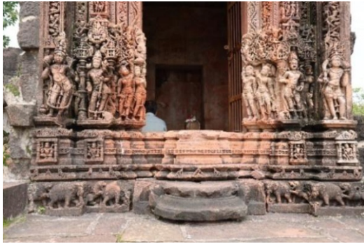
Figure 58 Lower section of the doorframe
